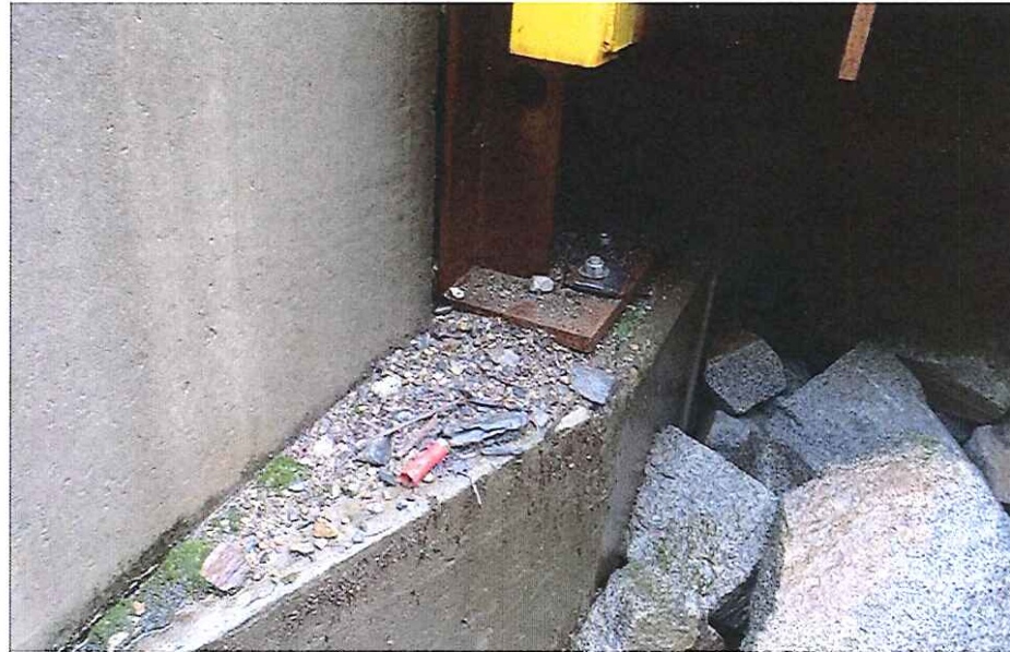
CK2442 Left Abutment Bearing
