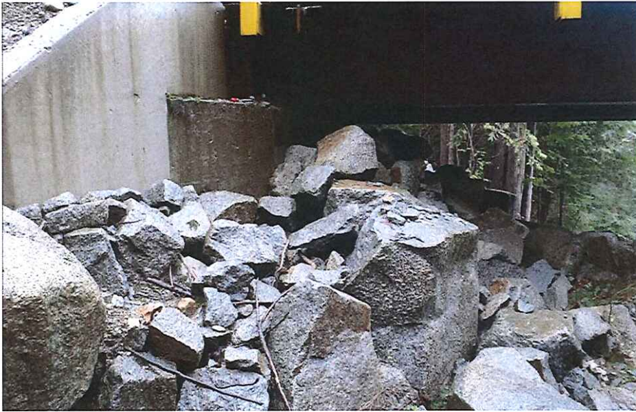
CK2442 Left Abutment
