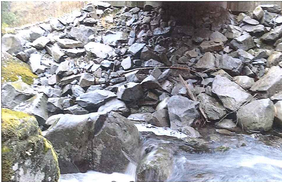
CK2442 Right Abutment
