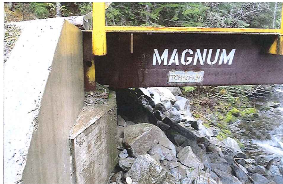
CK2442 Right Abutment bearing
